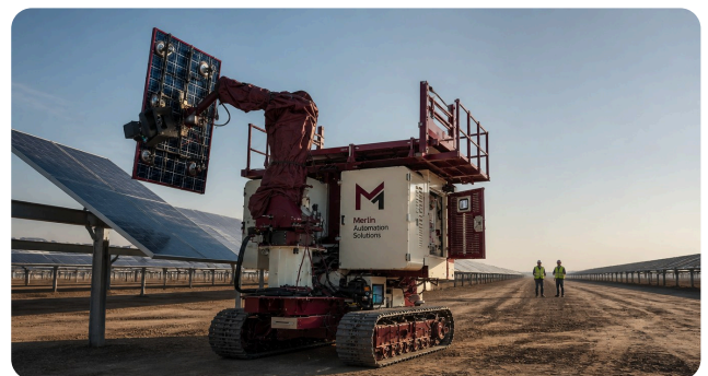
Crawler-mounted platform with robotic module gripper
